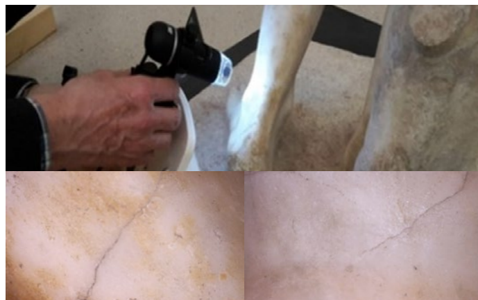
Figure 24: Small handheld digital microscope and detected cracks © Erich Jelen, Fraunhofer UMSICHT
