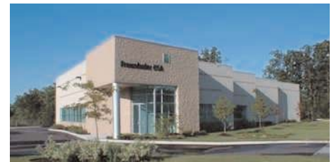
Building of CCL, CLT (Center for Laser Technology), and Fraunhofer USA Headquarters in Plymouth, Michigan
